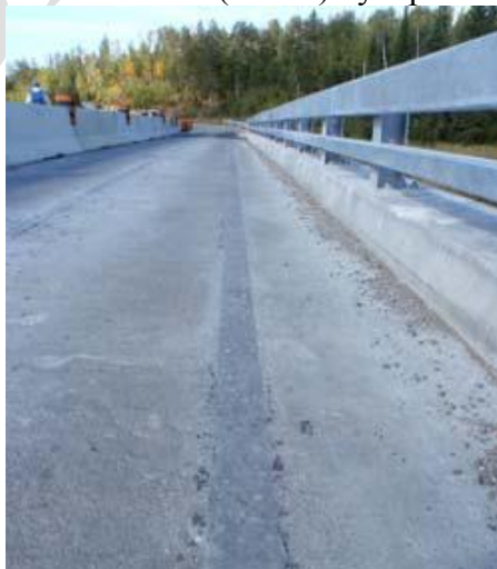
Obr. 20 The Log River Bridge, Ontario, Kanada, zdroj [65]
