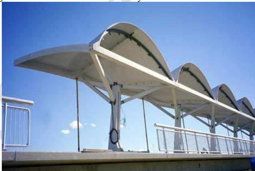
Obr. 34 Shawnessy Light Rail Transit Station (zdroj http://www.cpci.ca )
