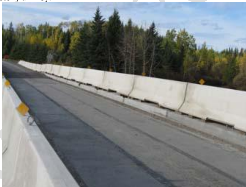
Obr. 17 The Sunshine Creek Bridge, Ontario, Kanada, zdroj [65]
