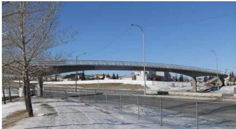
Obr. 18 The Country Hills Pedestrian Bridge, Alberta, Kanada, zdroj [3.1]
