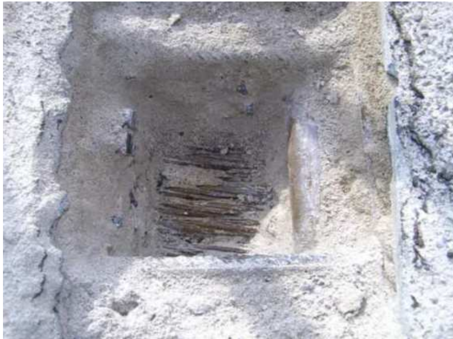
Obr. 14 Detail DT sondy [6]
